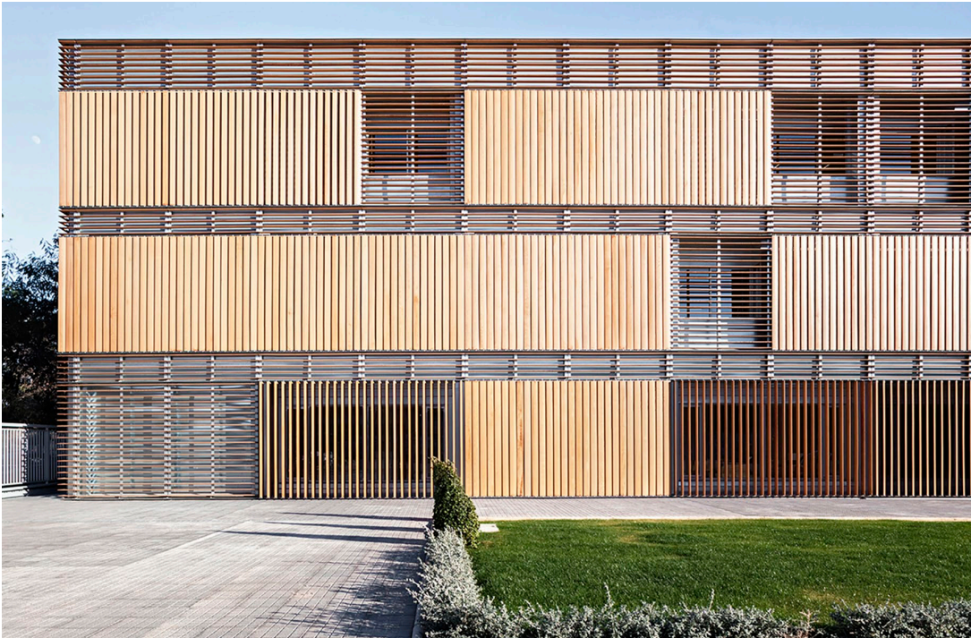
In the west block of the Centre d'Idiomes de la Universitat de València, Spain, by Arkitera SLP, the combination of fixed and movable sunshade slats defines the structure of the façade.
