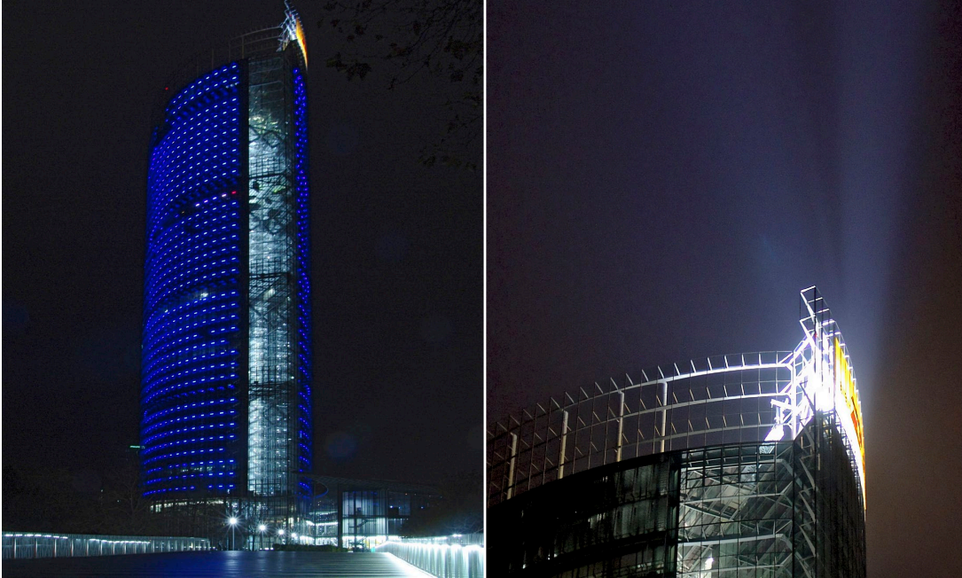
Effect lighting behind the outer glass façade and illuminated company logos on the roof lure migratory birds to their death at the Post Tower in Bonn. Exposed advertising panels, construction cranes, aviation safety lights, and other light sources high above the ground lie in the flight path of migratory birds and present an often-underestimated threat.
