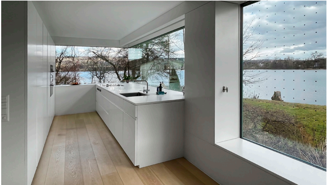
The glass industry is taking a growing interest in bird protection and is working with ornithological researchers to develop discreet and elegant markings. While detached houses frequently have high collision rates, there is often a high acceptance of markings in these cases. This highly effective dot grid was applied after construction.
