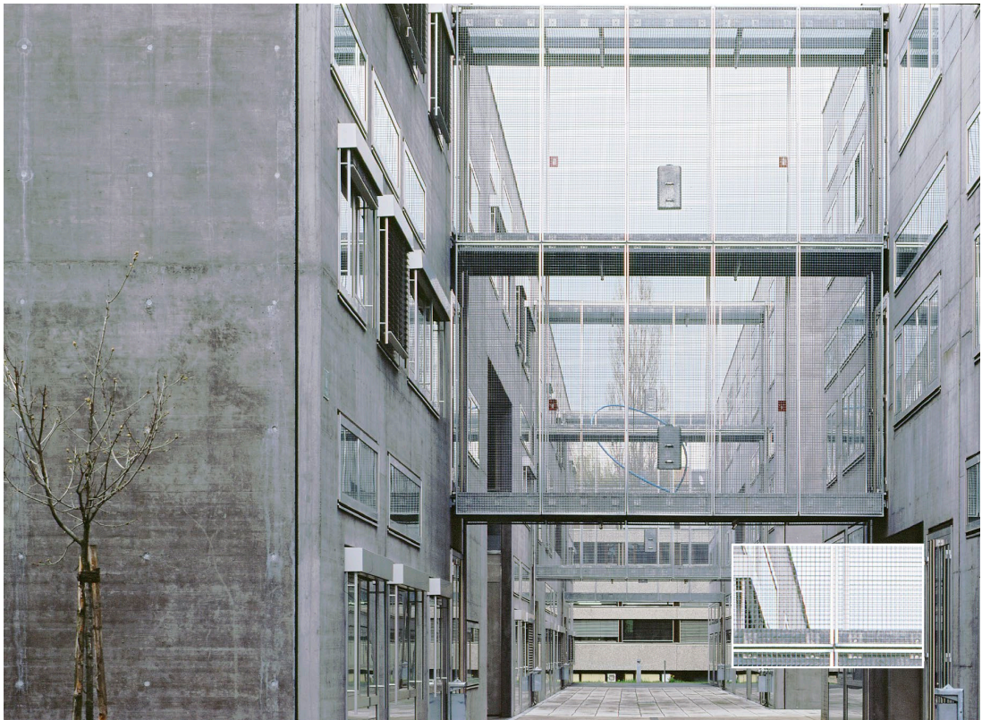
The individual buildings of the Graz University of Technology, Austria, by the architectural firm Riegler Riewe, are connected by multi-storey bridges. The façade elements made of steel lattice allow both transparency and the incidence of natural light, while remaining easily recognisable as an obstacle for birds.
