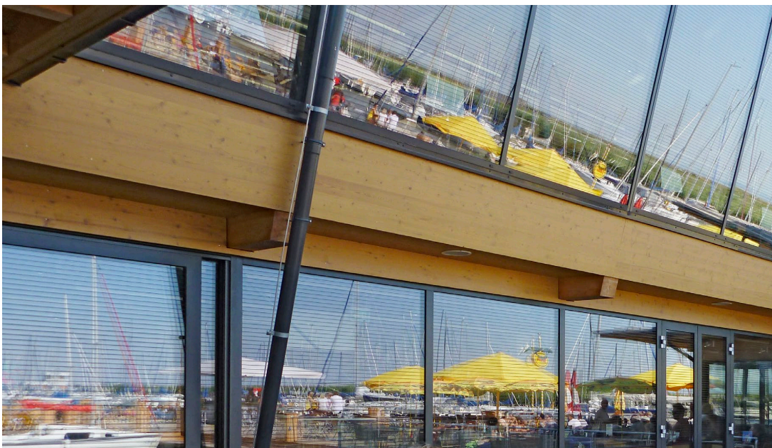
The window panes of this lakeside restaurant at the Neusiedler See National Park (Austria) were printed with thin black lines on the outside.
