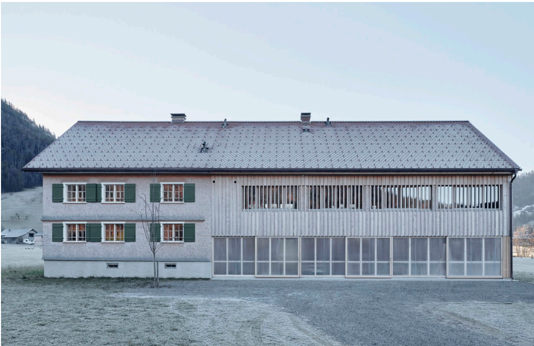
When renovating and repurposing the heritage building 'Großenbündt' in Hittisau, Austria, the architects Gruber Locher Architekten provided light to the ground floor by using semi-transparent materials. While the traditional grid windows of the residential wing were retained, the structure of the traditional wooden façade was echoed in the wooden slats over the long ribbon windows on the upper floor. Birds can easily recognise these materials and structures.
