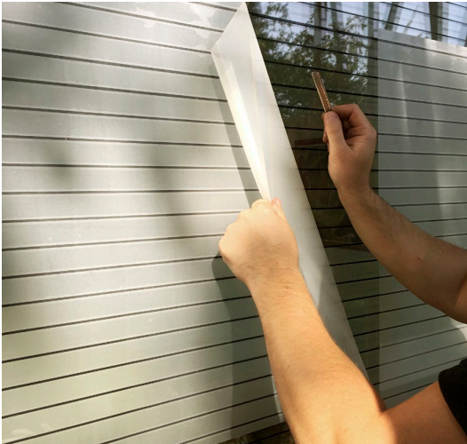
When plotted film patterns are applied, only the pattern elements themselves adhere to the glass.
