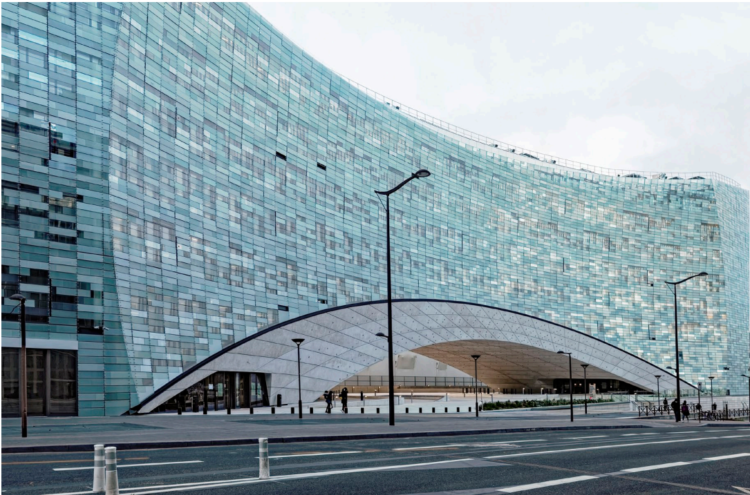
The façade of the headquarters of Le Monde in Paris, designed by Snohetta, is made up of more than 20,000 glass elements. These vary in structure and transparency and are arranged in such a way that they maximise the light in the offices and provide views to the outside in the right positions.
