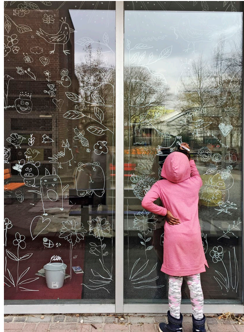
In this creative marking, the motifs are distributed over the entire surface without leaving any large gaps. Despite this, the view from inside is not greatly restricted and the windows continue to provide light.
