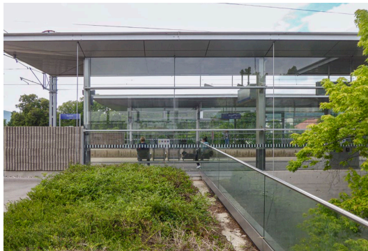
In green surroundings, glass structures like the entrance to this station are particularly dangerous for birds.
