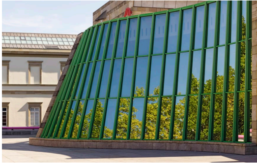
The smooth surface of glass casts reflections whenever the background is less illuminated than the foreground. Additional coatings on the glass façade can create higher-contrast reflections. For birds, the reflections of both trees and skies give the impression of open space.
