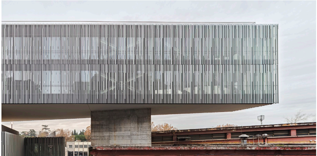
The Città del Sole ('Sun City') in Rome, by Labics, is a multipurpose facility with public and private functions. Both the design of the façade's aluminium panels and the translucent glass slats on the various buildings provide protection from the sun and for birds in equal measure.
