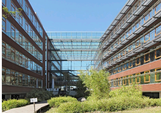
In green inner courtyards or areas of buildings which are enclosed from multiple sides, the risk of collision with glass surfaces increases. Vegetation attracts birds flying over the sea of buildings, but once they are inside they can have trouble taking off at a steep angle and flying away.
