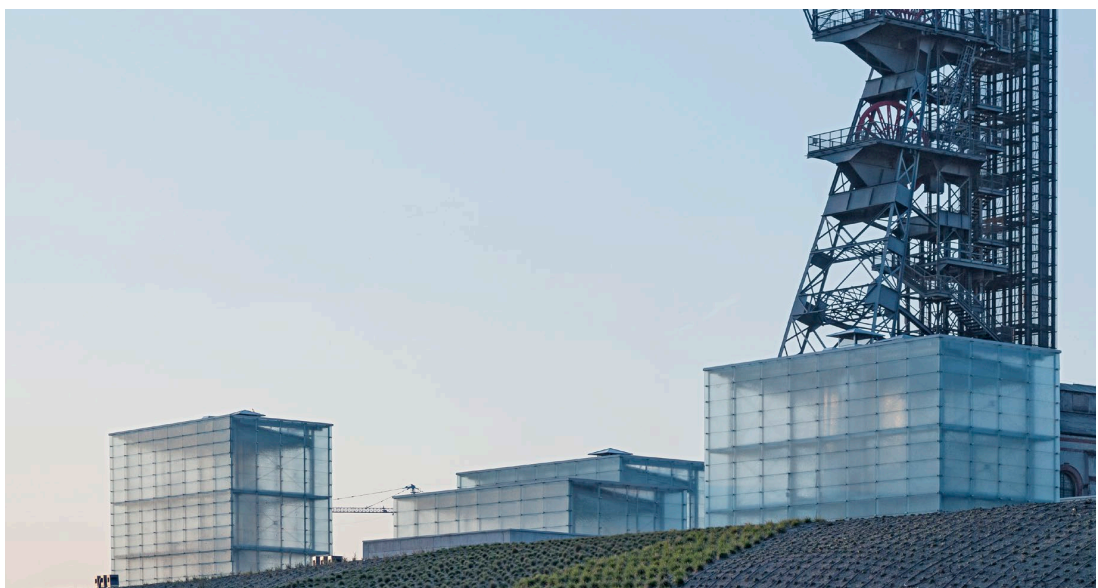
At the Silesian Museum in Katowice, cubes with a façade of etched glass provide the underground museum rooms with daylight. The abstract glass cubes by the architectural firm Riegler Riewe blend harmoniously into the ensemble of existing historical buildings.
