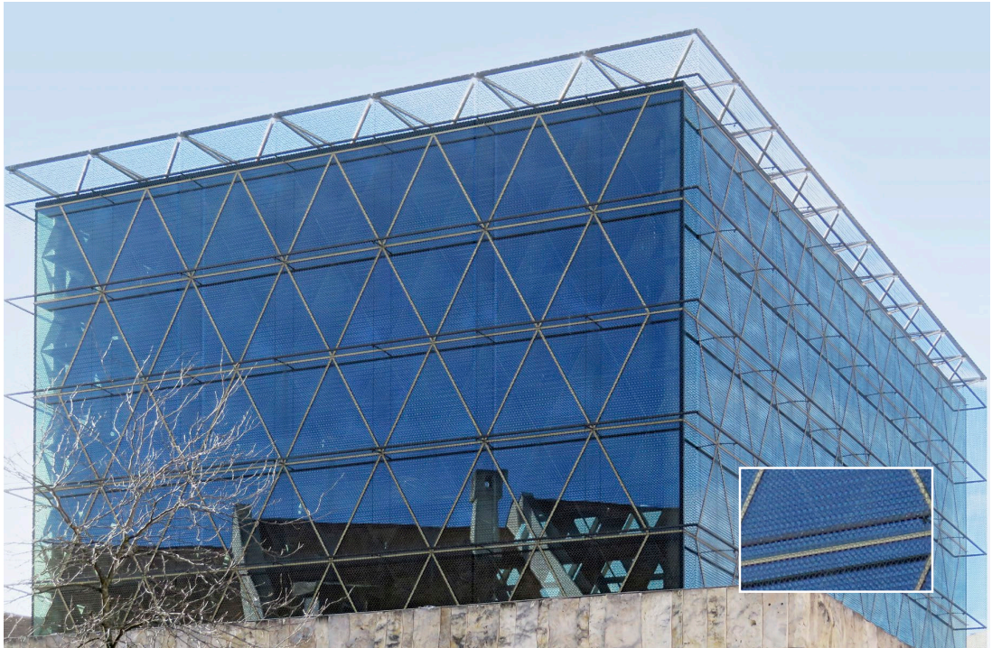
The glass cube of the Jewish Centre in Munich, by Wandel Hoefer Lorch + Hirsch, is surrounded by a steel structure and a bronze mesh. A triangular pattern of Stars of David creates a special atmosphere in the prayer room through the interplay of light and shadow.
