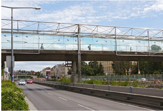
Glass windbreaks on bridges and connecting walkways are among the most conspicuous traps for birds. In many places, silhouettes of birds of prey have been stuck onto the glass. While these are ineffective, they confirm that collisions occur on these areas.
