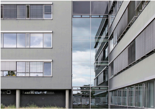
Birds perceive long strips of windows and reflective glass surfaces as opportunities to fly through the structure of the building. Individual subdivisions within glass surfaces do not reduce the risk of collision.
