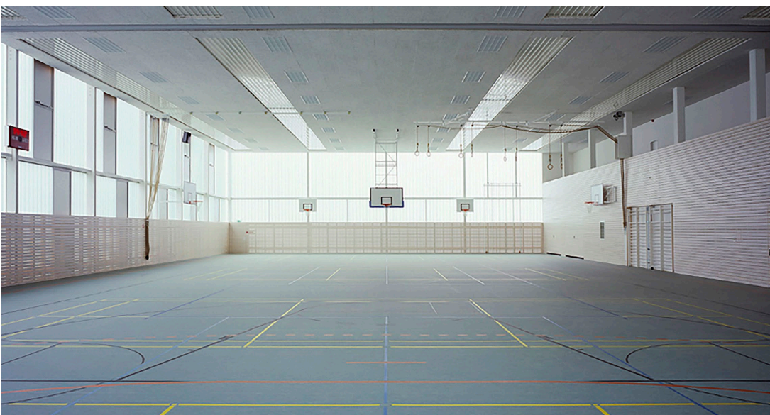
The building envelope of this ball sports complex in Ingolstadt, Germany, by Fink+Jocher, consists of a channel glass construction filled with translucent thermal insulation between its two glass profile shells. This enables sufficient light to enter without causing disruptive shadows on the court.
