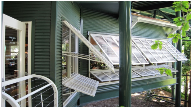
Shutters overhang windows at a facility at the San Diego Zoo. Photo by Christine Sheppard, ABC
