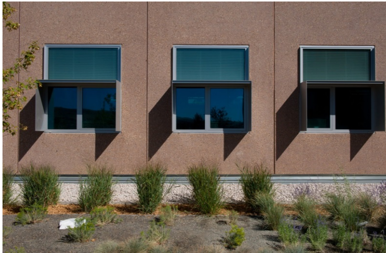
Shading was applied around the windows on the exterior of the Research Support Facility, National Renewable Energy Laboratory to reduce glare and overheating of the building interior. These windows are also bird friendly. Photo by Dennis Schroeder, NREL 19798
