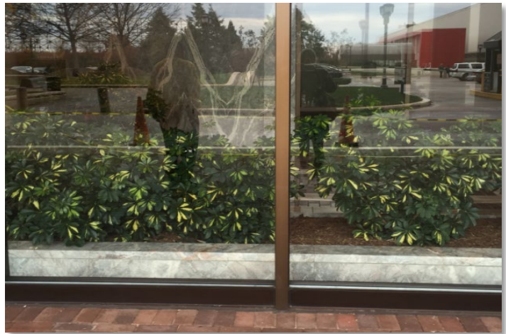
An example of where a potential bird hazard has been created by placing plants inside of a building near the window. Photo by USFWS
