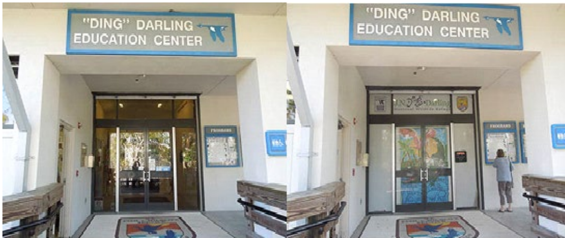
Bird friendly film was applied at the entrance of the Ding Darling Education Center at the J. N. "Ding" Darling National Wildlife Refuge. Photo shows entrance before (left) and after (right) application. Photos by USFWS
