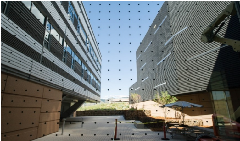
Dot pattern applied to the exterior of a National Renewable Energy Laboratory (NREL) building to help prevent bird collisions. Dots are approximately 1/2" in diameter spaced 2" vertically and horizontally. Photo by Dennis Schroeder, NREL 31193
